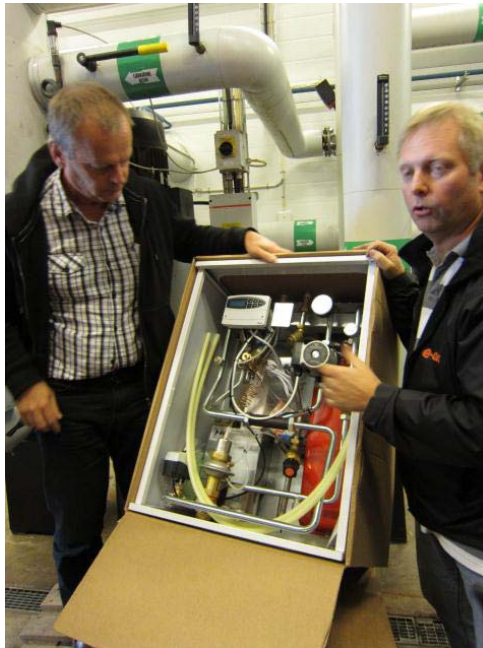
Heat Exchanger unit fitted into houses
